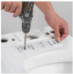
Install the screws from both sides
