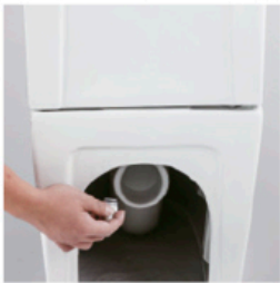
Install the screws and tighten them
