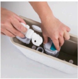
Install the water fill valve next
