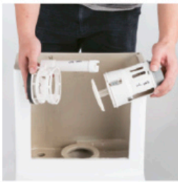
Disassemble the base of the outlet valve and flush bucket
