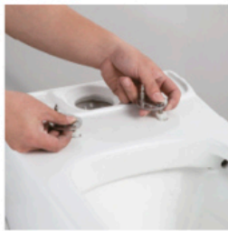
Install the slot on the toilet bowl
