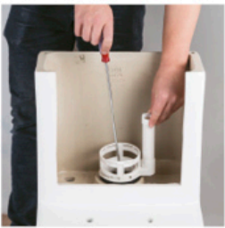
Tighten the water outlet valve base screw
