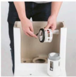
Loosen the water outlet valve base screw
