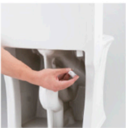
Tighten the screw of water inlet valve
