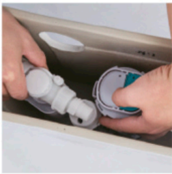
Place the water inlet pipe
