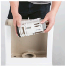
Install the water flush valve first
