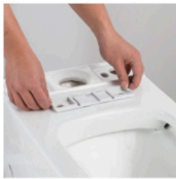
Align the slot at the hole in the toilet cover
