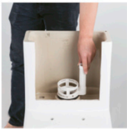
Tilt into the water outlet valve base
